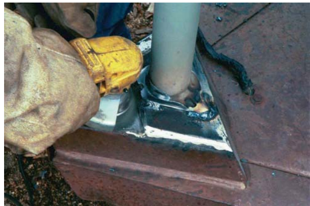
FIGURE 1-8 Angle grinding a weld to prepare it for finish painting. Larry Jeffus
