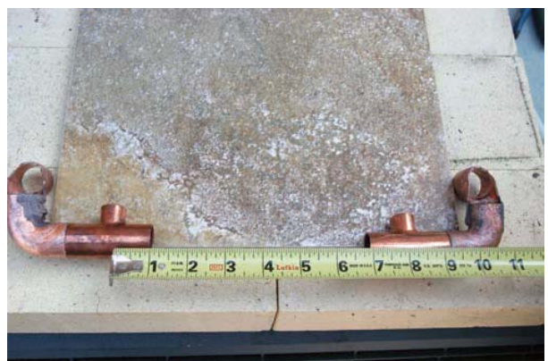
FIGURE 20-56 Lay the pipe on the tile to check the length of the copper pipe. Larry Jeffus
