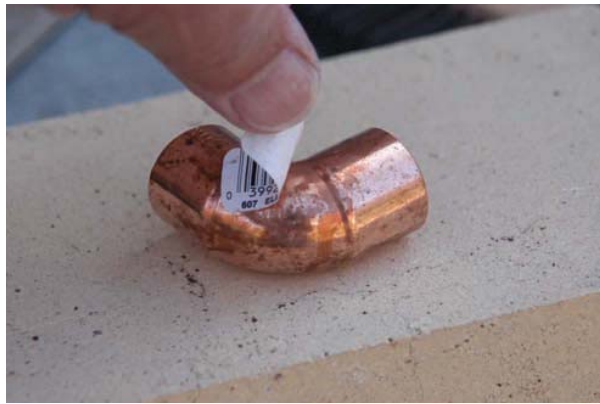
FIGURE 20-52 Peel off any stickers before soldering. Larry Jeffus
