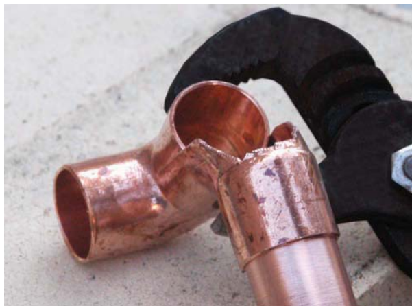
FIGURE 20-62 Hold the parts in place. Larry Jeffus
