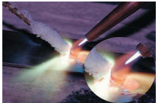
FIGURE 19-31 Deposit a spot of braze on the plate and continue heating the plate until the braze flows onto the surface. Larry Jeffus
