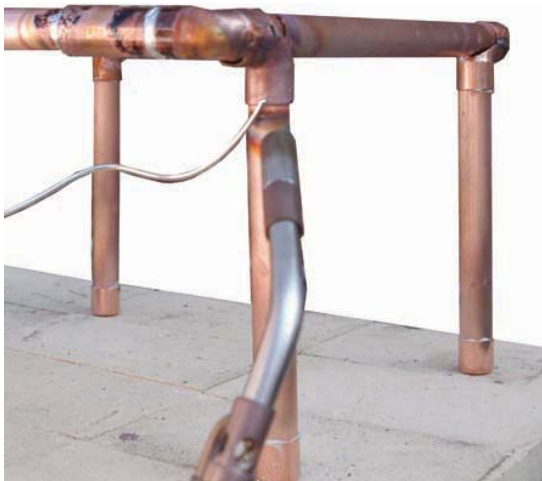
FIGURE 20-68 Solder the assembly in place. Larry Jeffus
