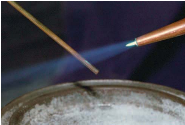
FIGURE 19-30A Heating a brazing rod. Larry Jeffus
