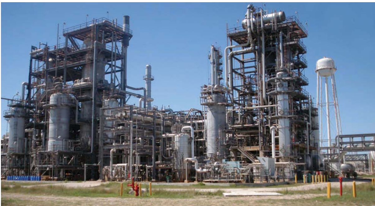
FIGURE 6-1 Petrol chemical refinery near Point Comfort, Texas, along the South Texas coast. Larry Jeffus
