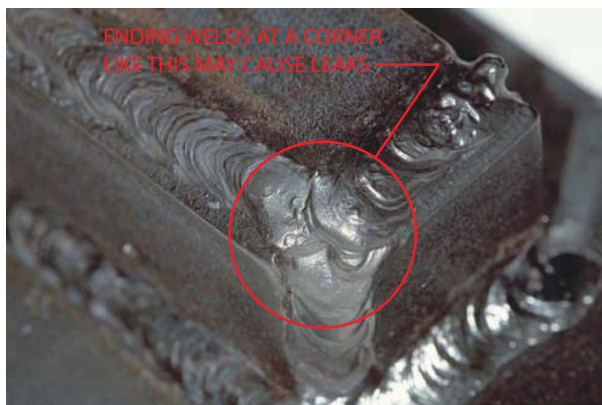
FIGURE 29-10 Incorrect method of welding a corner. Stopping on a corner like this may cause leaks. Larry Jeffus
