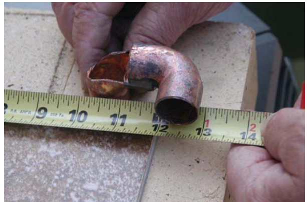
FIGURE 20-54 Use the tile and fitting to determine the length that the copper pipe should be. Larry Jeffus
